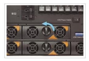
**STEP 4:** CE-R1 will display "communication fail" due to one module is inserted. Please enter the menu tree and change rectifier number to match latest rectifier quantity.
